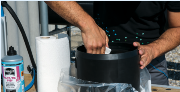
Clean the fusion zones of the fitting and pipe using a clean cloth.
