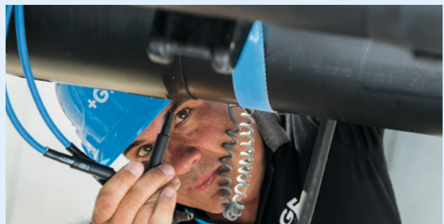
Connect the welding cables to the welding contacts of the fitting and weld according to the instruction manual.
