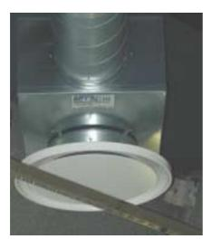
Figure 16. Plenum box connected to an air terminal device. Includes a regulating damper and acoustical cladding.
