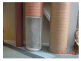
Figure 111 : Supply air register
