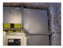
Figure 71 : Slip joints on a rectangular bend
