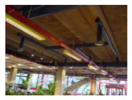
Figure 20 You don't always have to hide the ducts. Here false ceiling (seen to the left) has only been used where needed for acoustical reasons.
