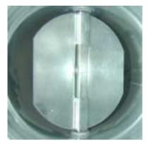
Figure 12 : Single-blade regulating damper. The blade angle can be manually adjusted or controlled with a motor.
