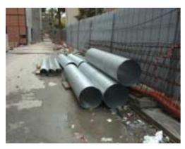
Figure 112 : Ducts exposed outside on construction site.
