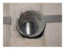
Figure 120 : Sharp screws increase the risk of injuries during maintenance operations
