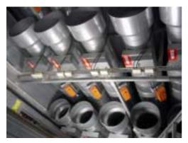
Figure 41 : Installation of vertical ducts in a high rise building in a space saving manner.
