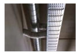
Figure 115 : Flexible duct
