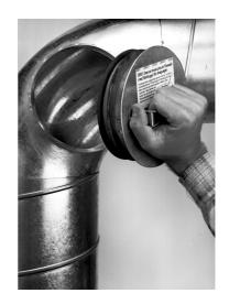
Figure 14: Bend with separate outlet for cleaning.
