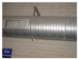
Figure 80 : Bracket-hanger for circular duct.
