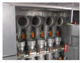
Figure 103: Ducts for the different floors pass down through common shafts, one for supply and one for extract air.
