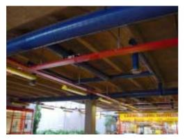
Figure 107 : Symmetrical design of the ducts results in the same pressure drop at each register
