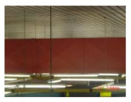
Figure 72 : Cross-bent duct sides to increase stability.
