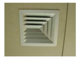
Figure 17. Rectangular supply air terminal device.
