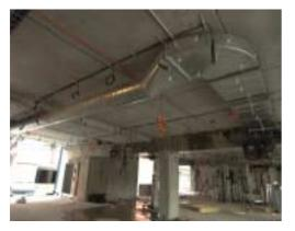
Figure 117 : Rectangular duct to be wrapped with insulation.
