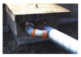
Figure 118 : Branching between a flexible and a rigid duct.
