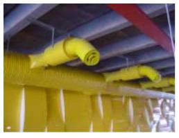
Figure 106 : Close-up view of supply air register with sound silencer
