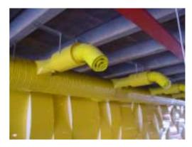
Figure 39 : Registers installed in parallel in a duct have to be provided with individual dampers, and perhaps also, as here, with silencers to reduce the noise from the dampers. Ducts (yellow) in a restaurant.
