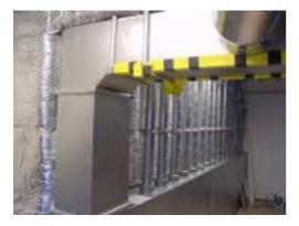
Figure 99: Rectangular ducts and plenums for supply (insulated) and extract air are connected to separate round ducts, one set for each exercise room. These ducts have manual airflow dampers.
