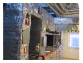
Figure 53 : Clean-out and inspection openings on vertical duct (left) and horizontal ducts.
