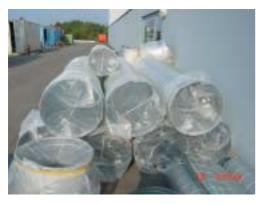
Figure 51 : Large ducts protected with end covers
