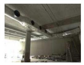
Figure 114 : Rectangular to circular reducer
